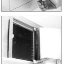
4. Bend over all of the dovetails on the frame with a hammer to ensure a tight fit.
