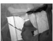
3. Remove the cover from the adhesive backed gasket tape.
