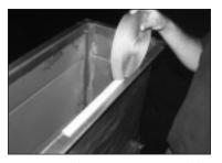
\*13A. System '45' requires 1" Ductmate 440 Gasket Tape. Start applying halfway between duct corners. Position on inside edge of Ductmate angle as in photo.
