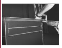
10. Work in one direction around duct when seating the frame. Fasten in sequence as you go. Do not fasten angle at corners first, it can cause seating problems.
