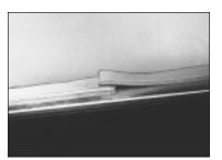
Apply 440 gasket completely around Ductmate frame to the beginning point. Where gasket meets overlay about 3/8".
