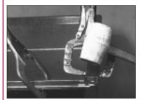
8. Use a mallet to seat the frame onto the duct. *Establish metal to metal contact along length of the angle.*
