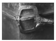
18. Compress gasket at corners with vice-grip while snapping in corner clips.
