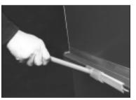
21. Ductmate 25/35 cleat can be snapped-on with the Cleater 1 Tool or with the Cleater II where space is restricted.
