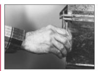
17. Carefully align mating frames before they touch. Ductmate 440 adheres on contact. A drift pin can be used to correct any misalignment.
