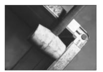
7. If the duct corner or the Pittsburgh lock gets caught under the Ductmate corner, tap the frame outwards to allow the duct corner to slide past the Ductmate corner piece. THIS IS VERY IMPORTANT!
