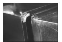
16. On the mating Ductmate frame apply 440 gasket only to the corners as in photo (approximately 3" per corner). The same 3 point application requirements apply as in photo 14.
