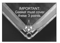
14. Position 440 Gasket in an arc so that it covers the three points in the duct corner. *Gasket must cover all three points.* Some gasket will protrude into the airstream. Press gasket firmly into contact with the raw edge of the duct corner and Ductmate corner assembly. Ductmate 440 is the preferred gasket. Refer to procedures on the back of the brochure for applications using Ductmate Neoprene Gasket.
