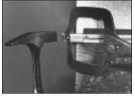
Slide corner clips onto the Ductmate 25/35 joined corner pieces. Tap with hammer until rear tab clicks into notch on corner pieces and locks in for a permanent connection.
